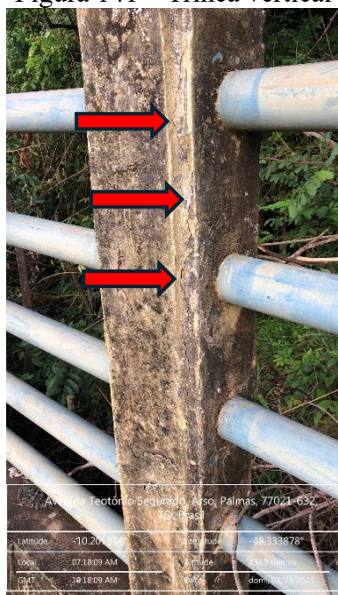
Figura 141 – Trinca vertical
